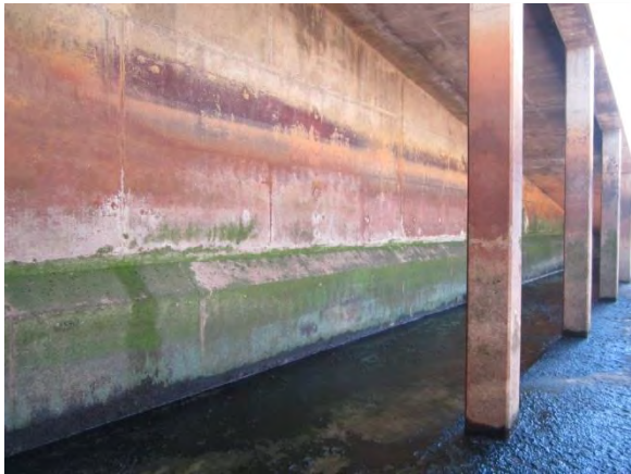
Photo 3-3. East wall of West FEB below ramp.
