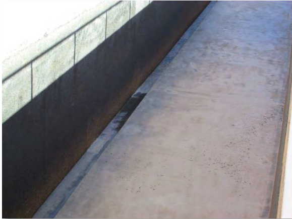
Photo A-68. General coating condition in south pass.
