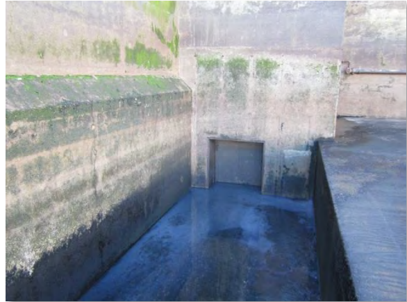
Photo A-49. Southeast corner of West FEB.
