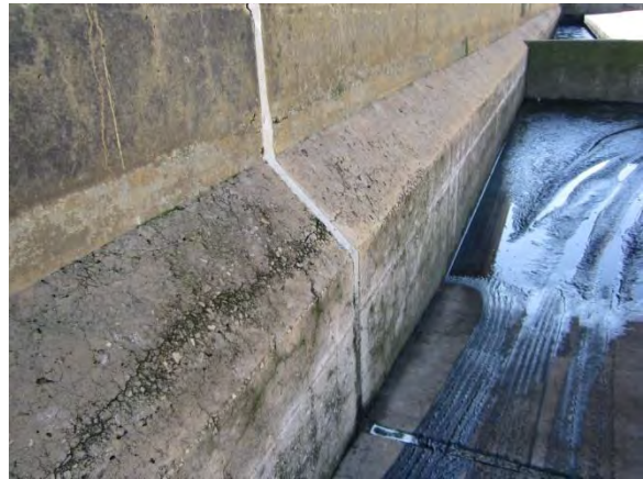
Photo A-57. Typical view of lower east wall.
