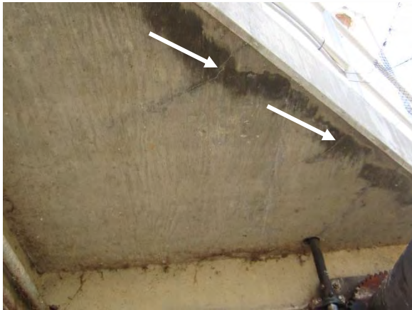
Photo A-41. Minor cracking on underside of diagonal platform over southeast corner of SST 2.
