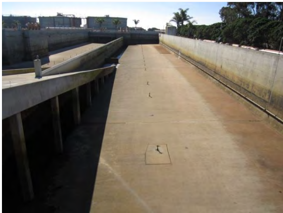
Photo 3-1. West FEB as viewed from platform at north end.
