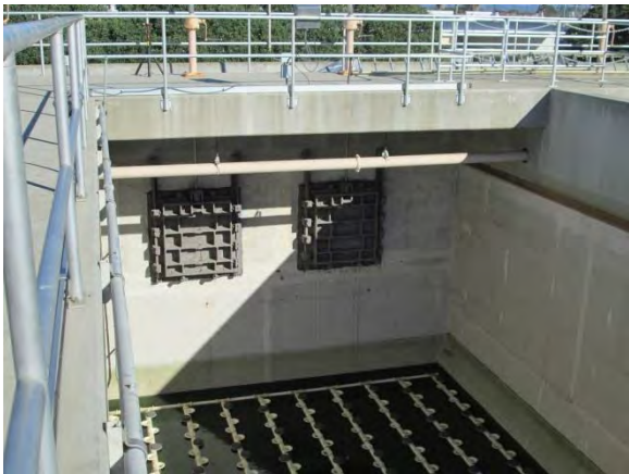
Photo A-3. North wall of AST 1B.
