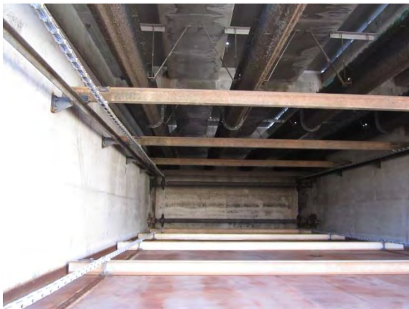
Photo 3-31. Looking west inside SST 2.
