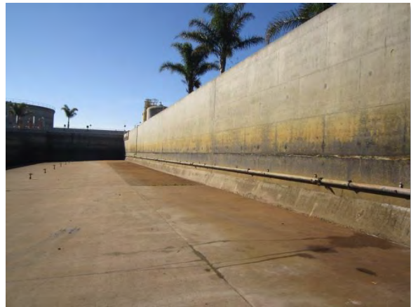
Photo 3-2. West wall near midpoint of West FEB.
