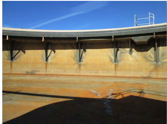
Photo A-20. General view of launders and wall inside PC 1.
