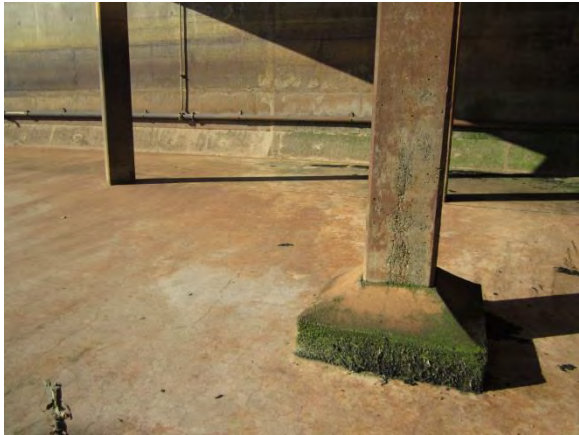
Photo 3-24. Columns at north end of West FEB.
