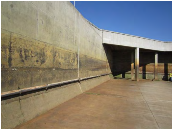
Photo A-50. Northwest corner of West FEB.
