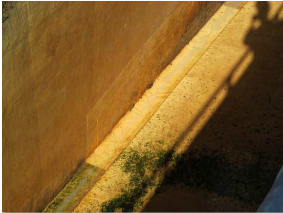
Photo A-75. Typical coating patch.
