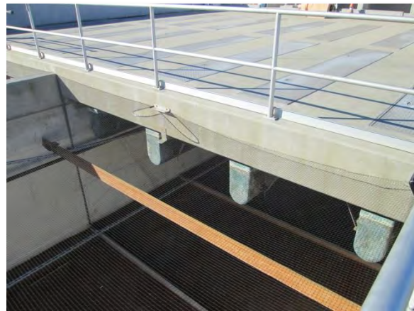
Photo 3-32. Platform and launders over west end of SST 2.
