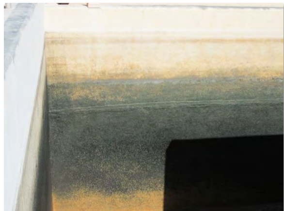
Photo A-78. Typical coating texture.
