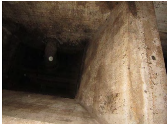
Photo A-36. Sump at southwest corner of SST 2.
