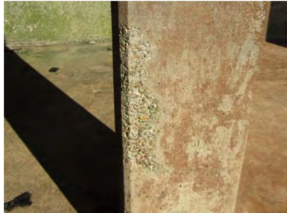
Photo 3-25. Typical exposed aggregate on column.
