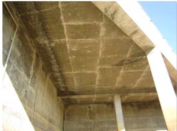
Photo A-51. Northwest corner of West FEB.
