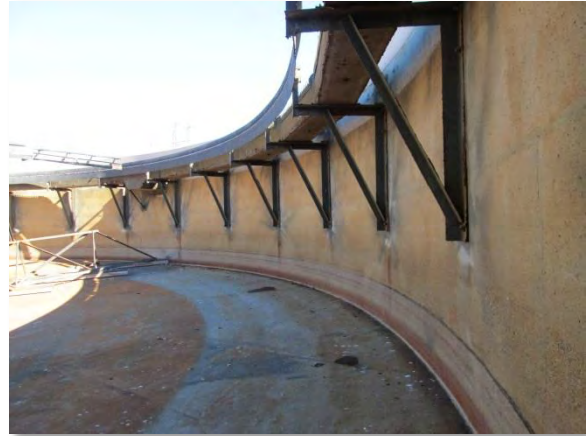
Photo 3-57. General view of launders and wall inside PC 1.
