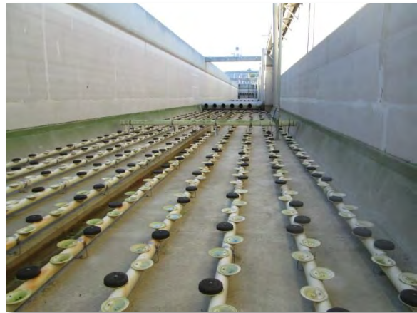
Photo 3-41. Looking south from north end of AST 1B.
