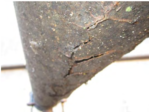
Photo A-66. Underside of horizontal pipe near south wall.
