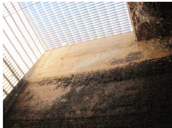
Photo 3-85. Coated surfaces above the outlet sluice gate were in good condition.
