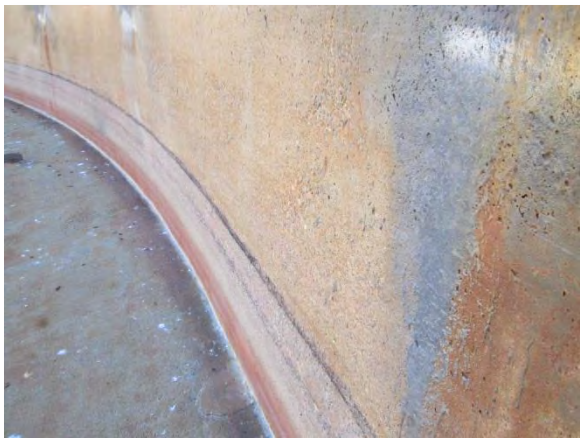
Photo A-23. Typical exposed aggregate on lower wall.
