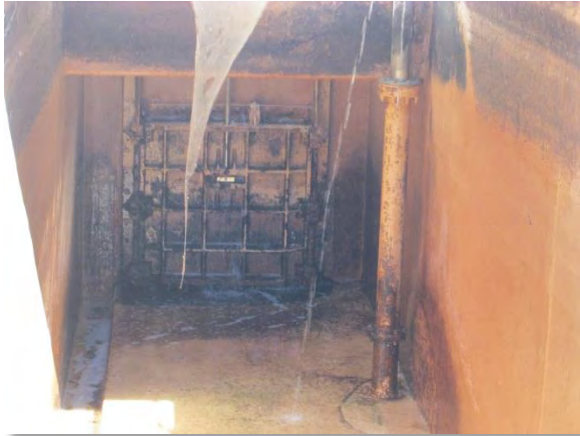
Photo A-72. Northeast corner and sluice gate.
