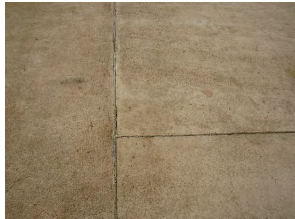
Photo 3-10. Typical control joints in floor.
