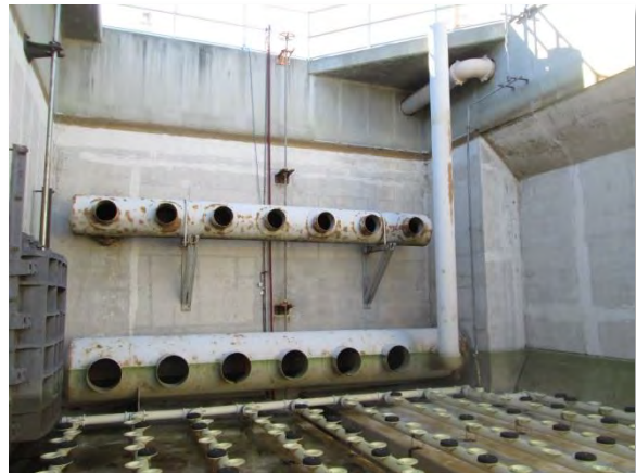
Photo A-4. South wall of AST 1B.
