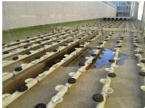
Photo 3-53. Puddle of water caused by groundwater infiltration at expansion joint 210 feet south of north wall.
