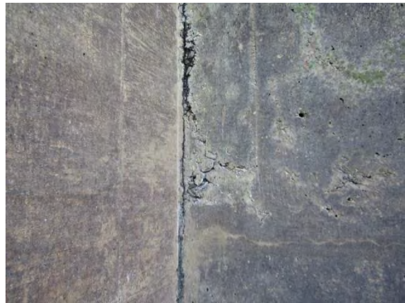
Photo A-59. Detail of southwest corner of West FEB.
