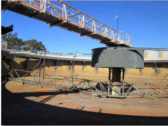
Photo 3-56. General view inside PC 1.
