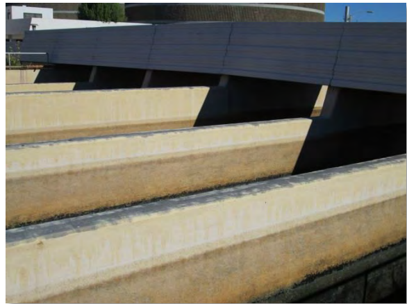
Photo A-71. General coating condition on upper walls.
