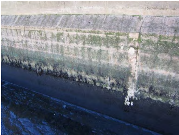
Photo A-56. Typical view of lower east wall.
