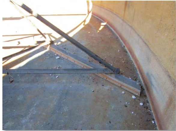
Photo A-30. End of rake arm within PC 1.
