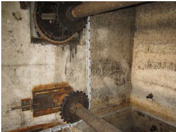
Photo A-35. Southwest corner of SST 2, above sump.
