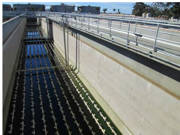
Photo 3-43. West wall of AST 1B (typical).
