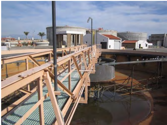
Photo A-19. General view of PC 1.
