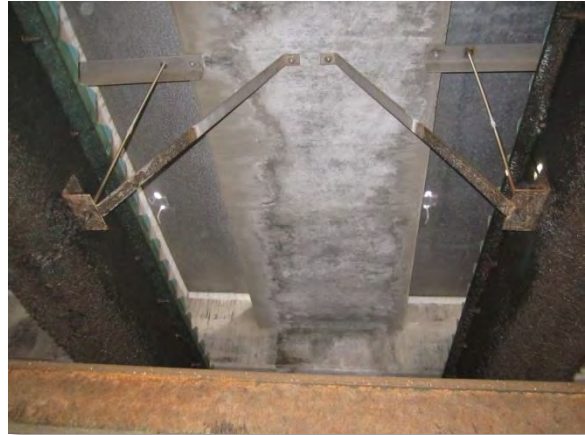
Photo A-34. Underside of platform at west end of SST 2.
