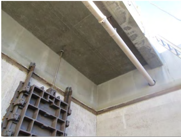
Photo A-5. Underside of platform at north end of AST 1B.
