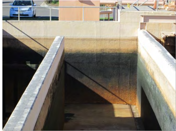
Photo A-69. General view of west wall from center pass.
