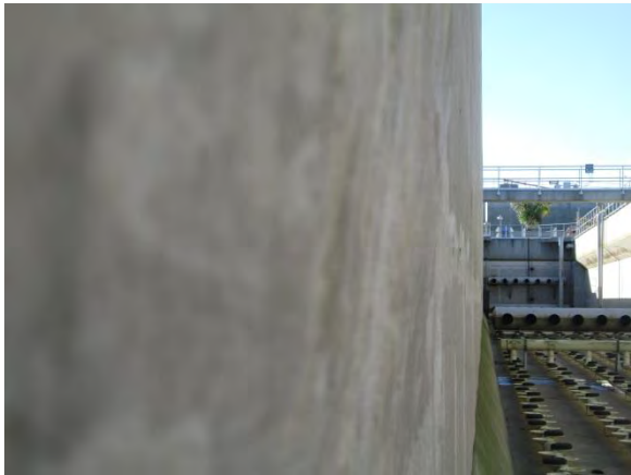
Photo A-13. Uneven construction joint (approx. 1-inch offset) on east wall about 150 feet south of north wall.
