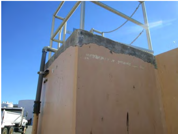
Photo C-9. Broken concrete at top of effluent tower (repaired).
