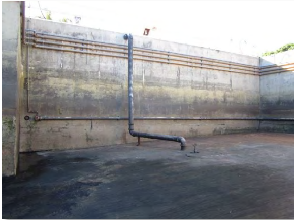
Photo A-48. South wall of West FEB.
