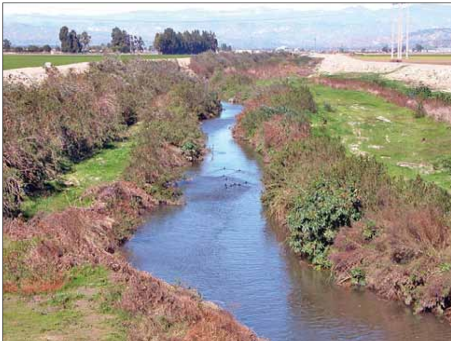
VIEW: Motorist's view of Revolon Channel.
