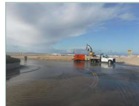
Coastal flooding at 5th Street and Mandalay Beach Road
