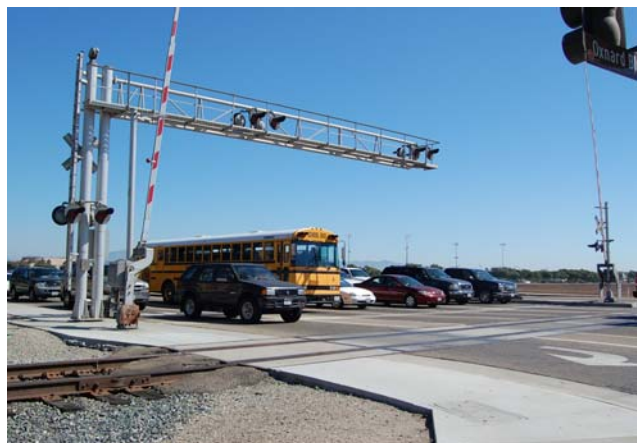
Intersection of Gonzalez Road at Oxnard Boulevard.
