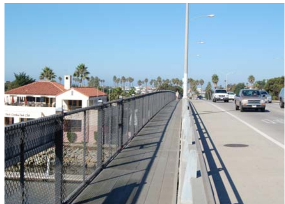
Pedestrian bridge on West Channel Islands Boulevard.
