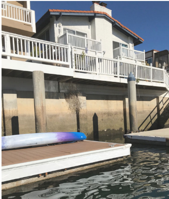
Figure 10 - Typical overhanging decks
