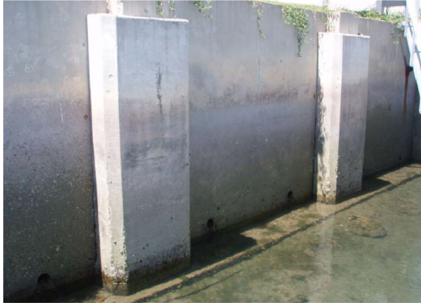
Figure 3 - Typical pilaster jacket repairs [from TranSystems (2017)]
