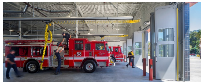
Figure 3 – Fire Station No. 8, City of Oxnard
