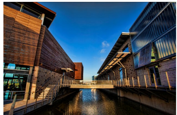
Figure 5 – Advanced Water Purification Facility, Oxnard
