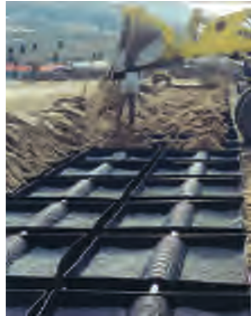
Stormwater Detention Beneath Park
