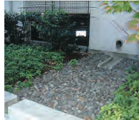
Bio-Retention Used with Roof Drains
