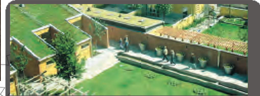
Green roofs on buildings and parking structures provide additional runoff collection and treatment areas
