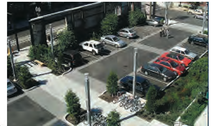
Parking lot landscaping can be used as stormwater collection and treatment areas
