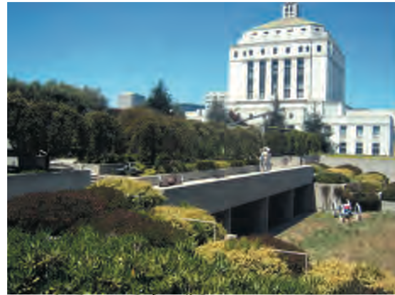
Green roofs on buildings and parking structures provide additional runoff collection and treatment areas
