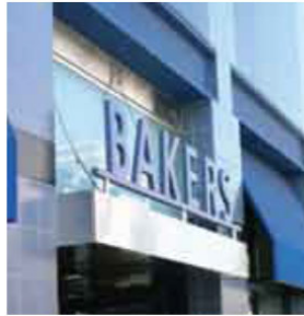
SIGNAGE SITTING ON STEEL CANOPY
